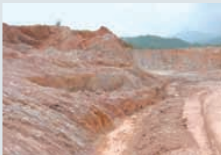
Large-scale earth works without erosion control BMPs
