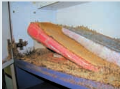
01 A kitchen cabinet badly infested with termites
