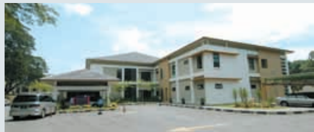
The newly established Sejahtera Centre
