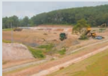
Large-scale earth works without erosion control BMPs
